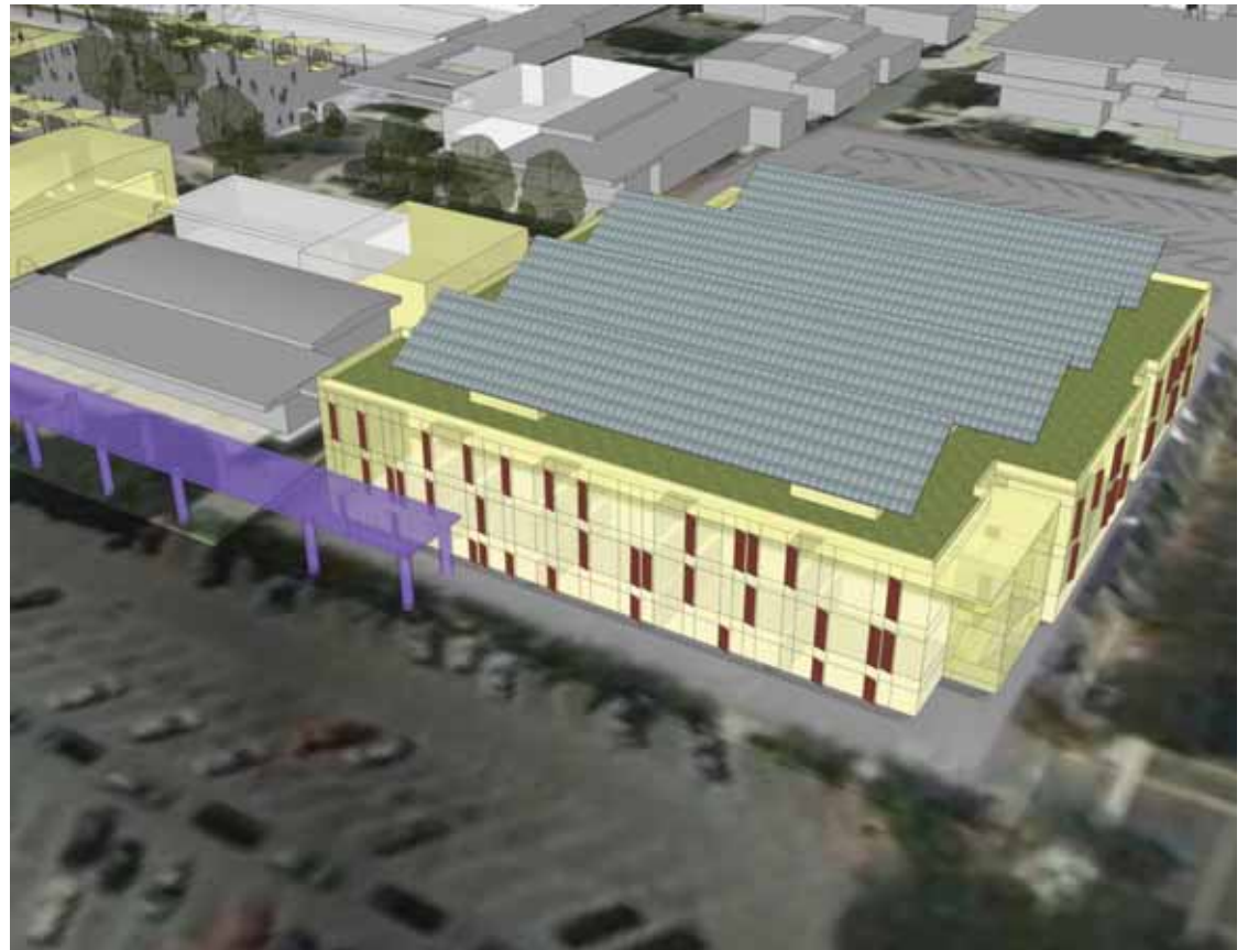
View from the southeast
